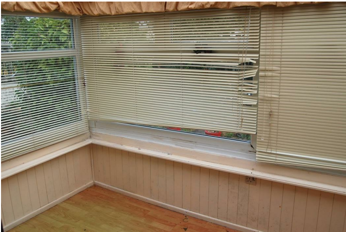
Timber cladding, partial upvc double glazing, timber door to side.
